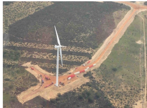
Figure 1. Typical wind turbine after installation.
