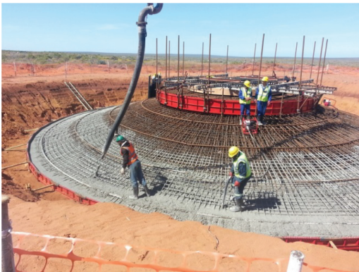
Figure 2. Casting of typical turbine foundation.
